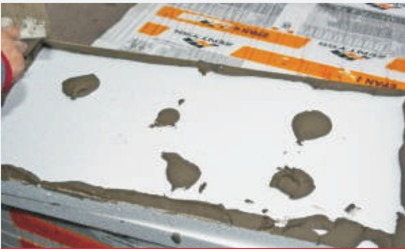
Applying adhesive to polystyrene boards
