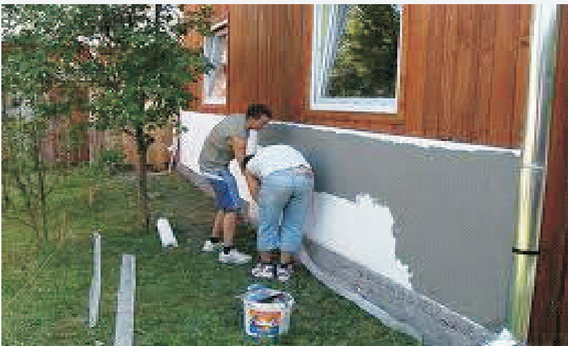
Applying base coat on polystyrene
