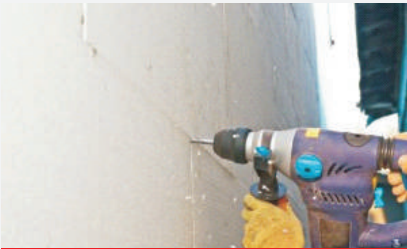
Drilling in concrete to fix polystyrene sheets
