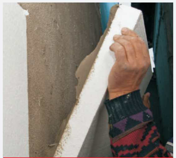
Attaching the polystyrene sheet to wall
