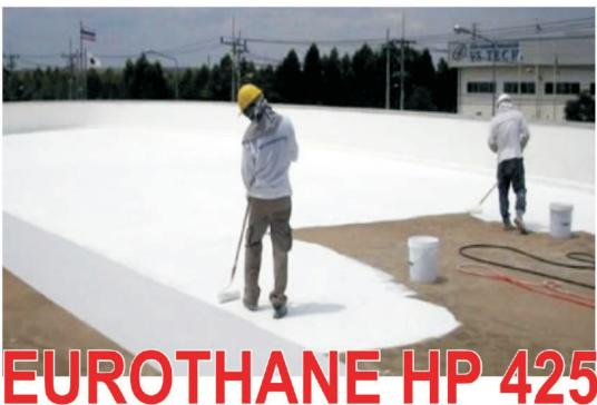
**Hybrid Polyurethane Liquid Applied Waterproofing**
